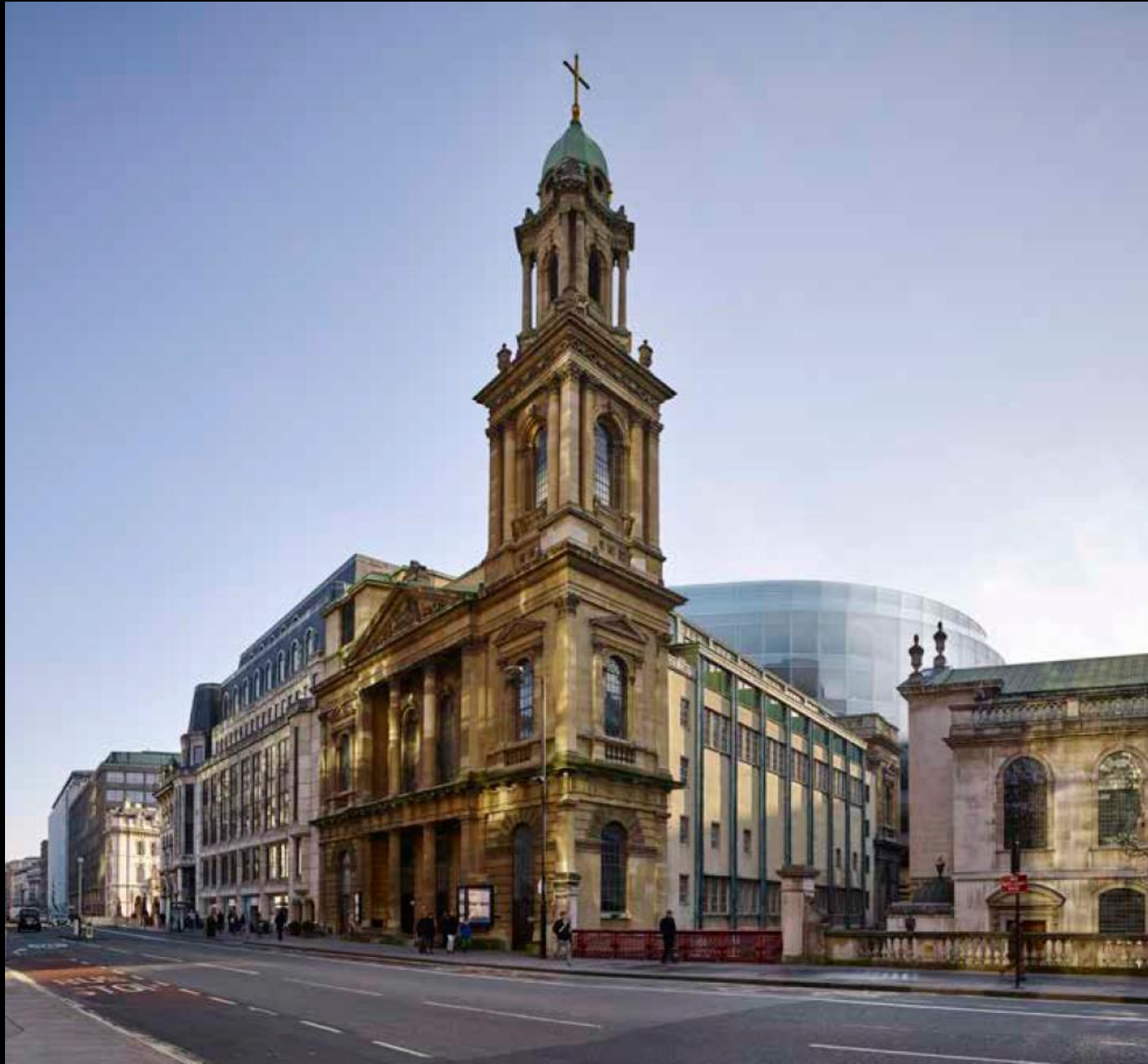
Existing view from Shoe Lane
